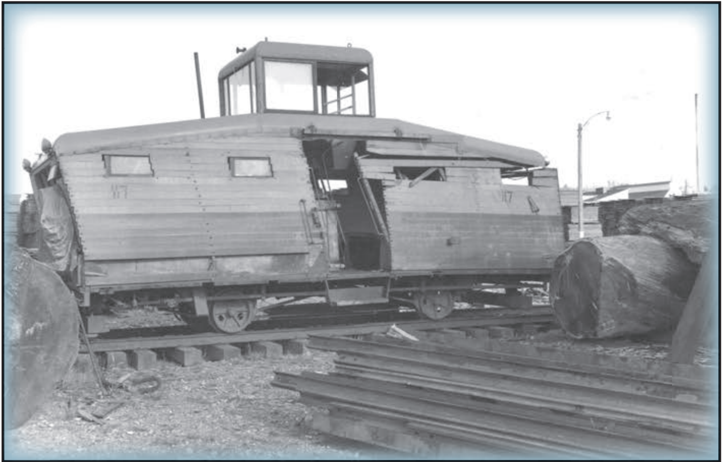
Above: This Simpson cupola type speeder had a head on collision with a gravel train in 1948. Photo, Simpson Archives.
