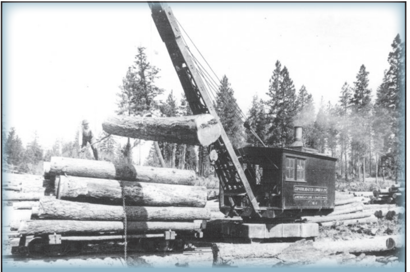
Below: Crane #4, an American Hoist and Derrick model D loader. Photo, John Cummings collection.
