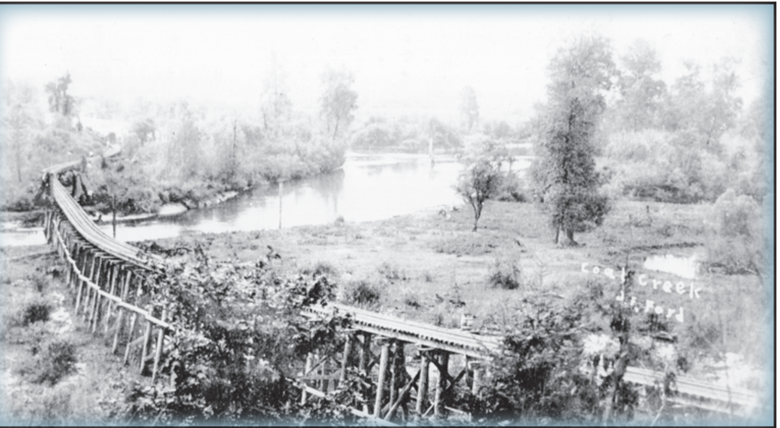
Above: A trestle and bridge over Coal Creek to the log dump. Photo by R. Reid, John Labbe collection.
