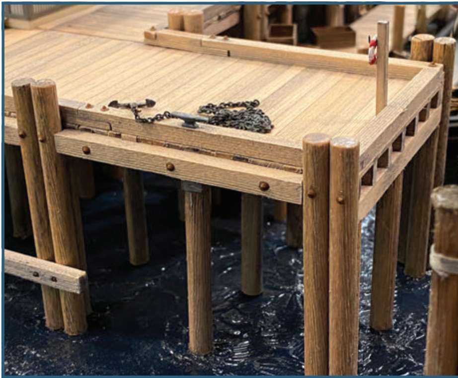
Left: The dock design is based on a Howard Fogg painting (see text). The pilings are 14-inch diameter posts. They are capped with a 13- x 13-inch-square beam. The stringers are 4 x 12s which in turn support the 3- x 10-inch decking. The guard beam on the top edge of the decking is a 10 x 10. The beam running between the pilings is a 12 x 12.
