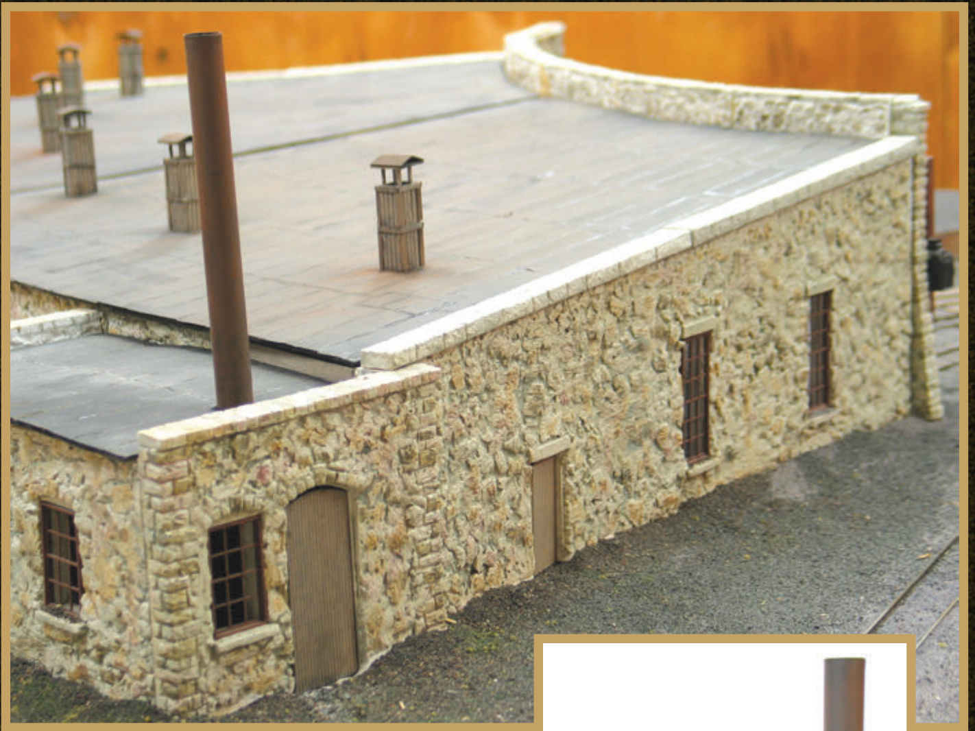
Above: Left side showing the boiler house addition.
