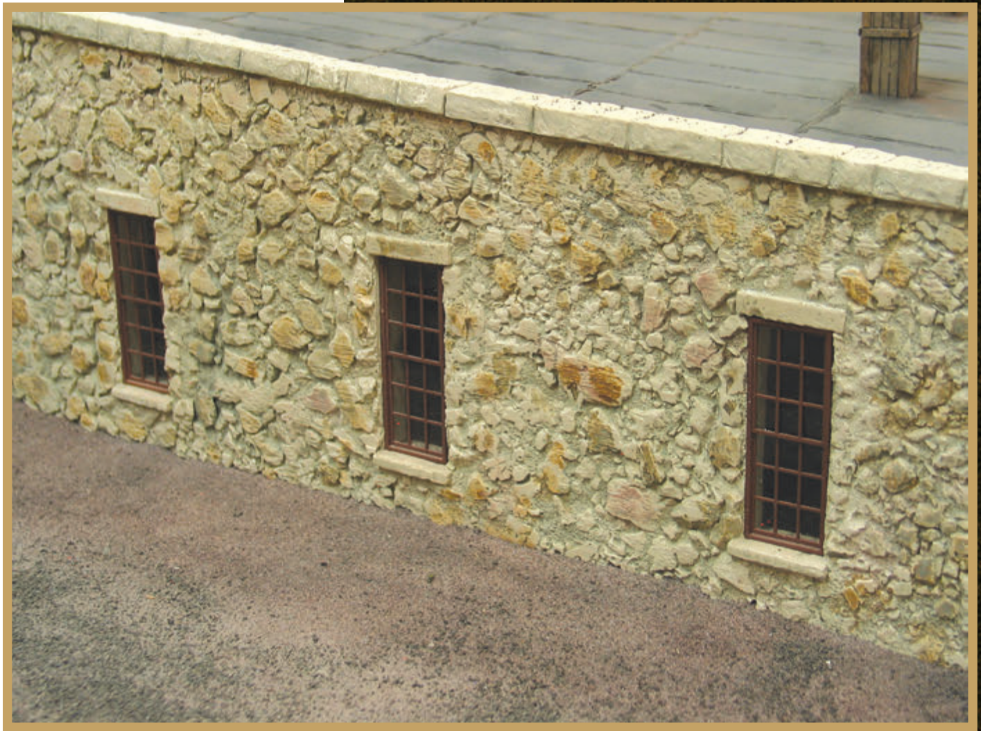
Above: The right side wall clearly shows the results of grinding down the original oversized stones with rotary rasps.
