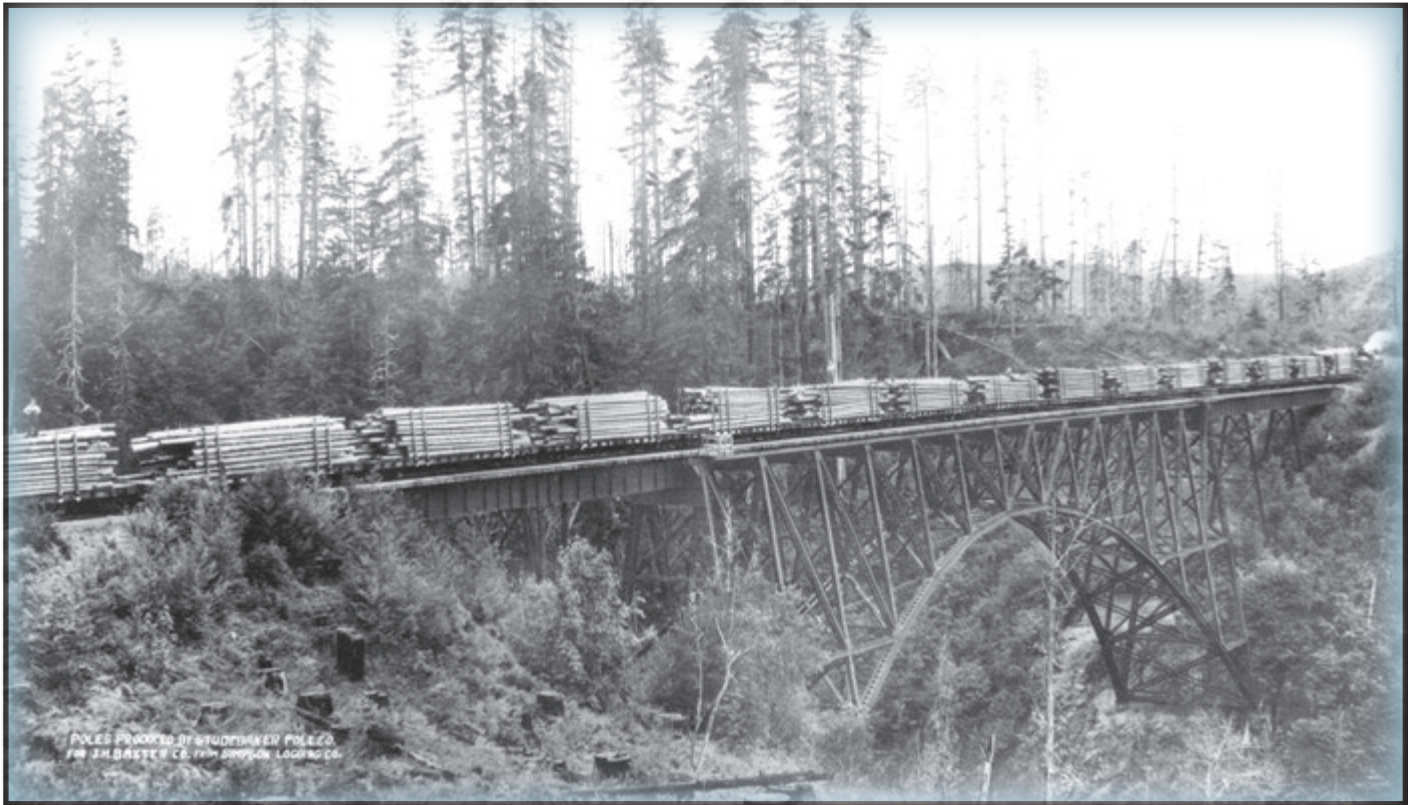
Above: The second canyon to be crossed on the new branch line was the South Fork of the Skokomish River that was quite a bit shorter, but somewhat higher than the Vance Creek bridge. It was constructed in 1929 and is shown here with a train loaded with poles pulled by 2-8-2 #11.
